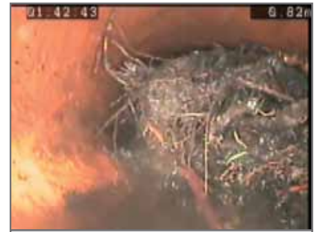
Fig 1.5 – 13.45m = Mass Roots 95% cross sectional area loss
